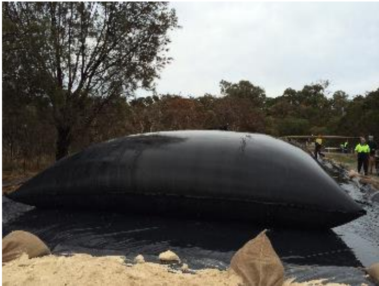
Figure 5.8 Using dewatering bags with MBOs at the Peel-Harvey Estuary, Western Australia.
